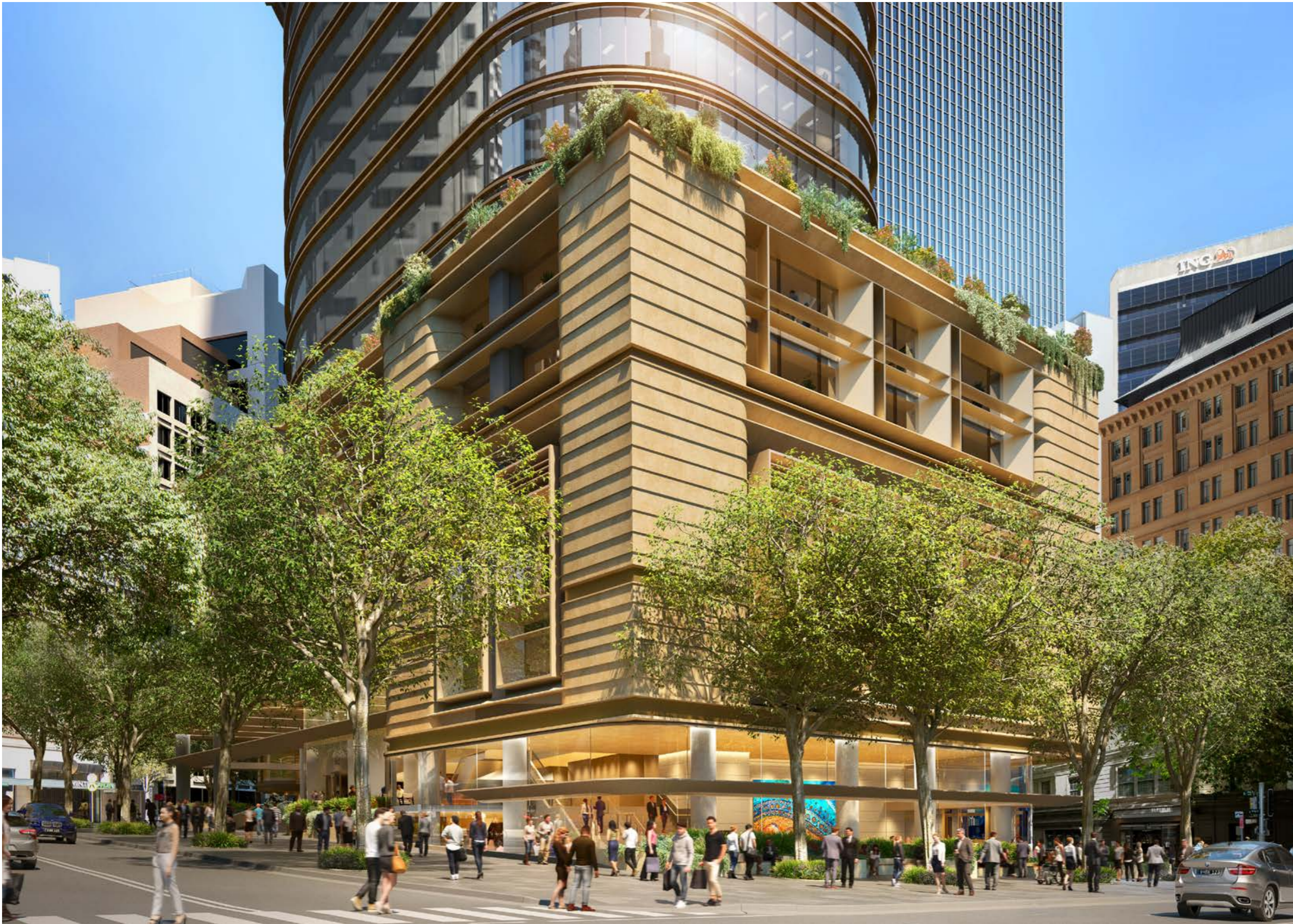
Bridge St Plaza view from Bridge/Gresham St
